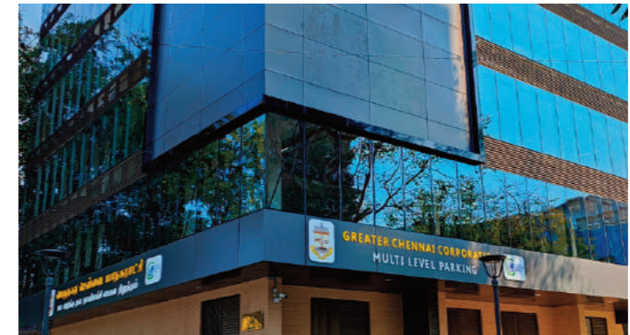
The GCC's seven-storey multi-level parking in T. Nagar
