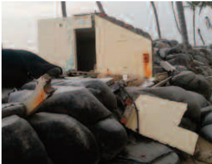
Remnants of a house destroyed by the raging sea
