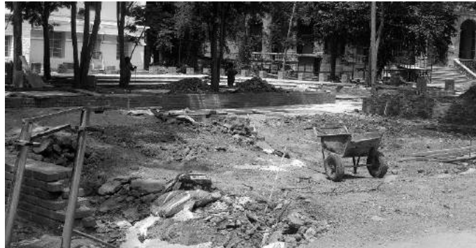
Construction work at the Government Museum
