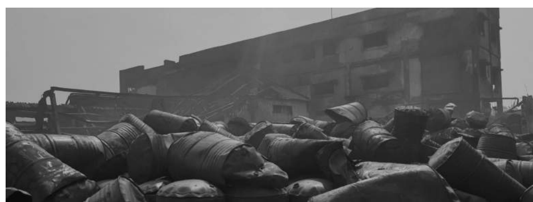
Burnt warehouse at Madhavaram | NEIL CORNELIUS
