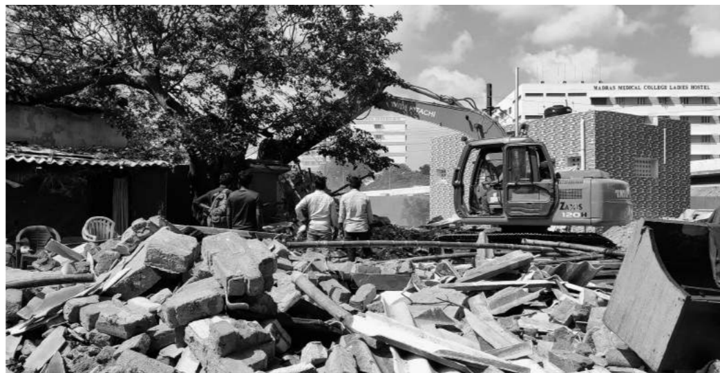
A bulldozer ramming down the houses at Sathyavani Muthu Nagar |
