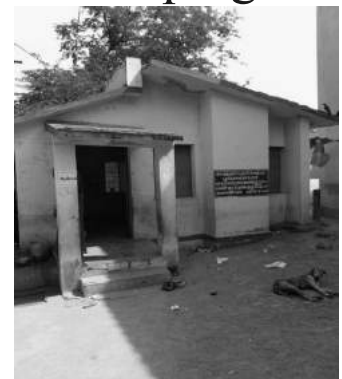
A temporary shelter for an anganwadi | ANMOL ARORA
