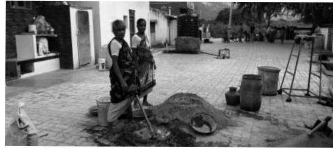
Vellaiyamma and Rajamma building toilets under MGNREGS | SHREYA HARIDAS
