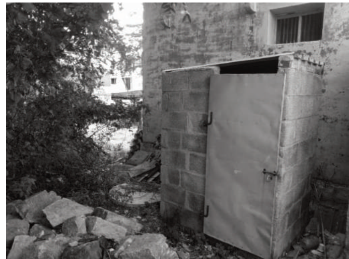
A toilet built adjacent to a house, under SBM | ANMOL ARORA
