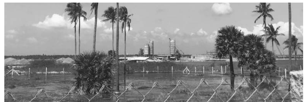
Under-construction Udangudi power plant
