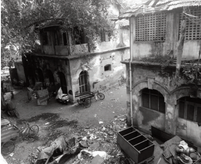
Dilapidated structures on government property on Davidson Street in George Town | ASHMITA MUKHERJEE
