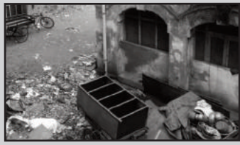
George Town buildings in disrepair Page 2
