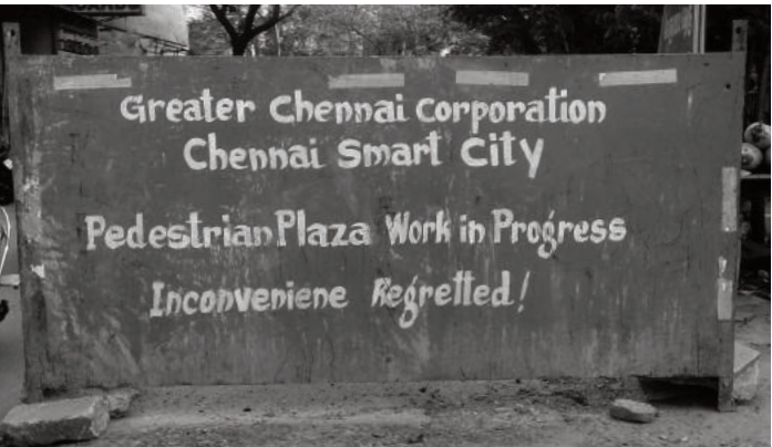
Construction ongoing at Pondy Bazaar | AKSHARA SRIVASTAVA
