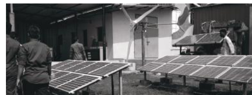
The station consists of solar trackers with three radiation sensors. AYESHA ROY
