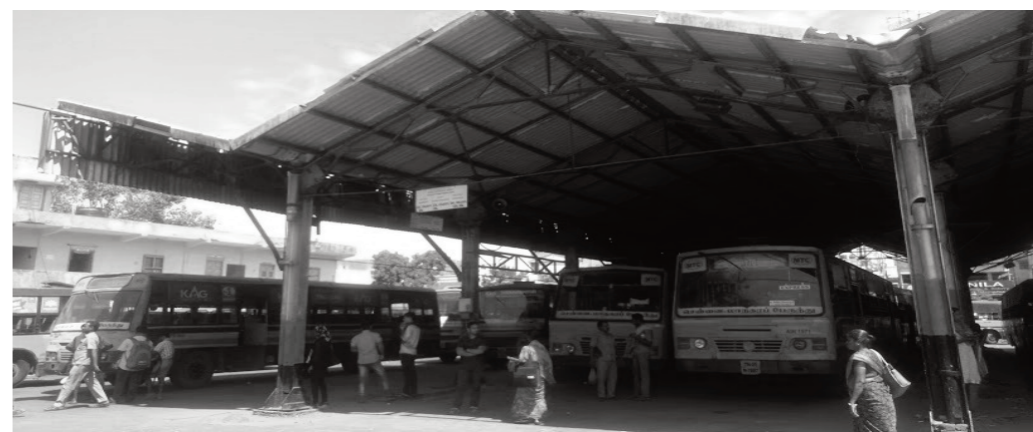
The Thiruvanniyur bus depot
