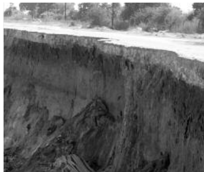
Landslides caused by blasting at the KPCL-EMTA coal mines in Baranj village | AIHIK SUR
