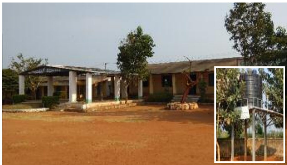
The first school in H. D. Kote to install solar-powered water supply system.
