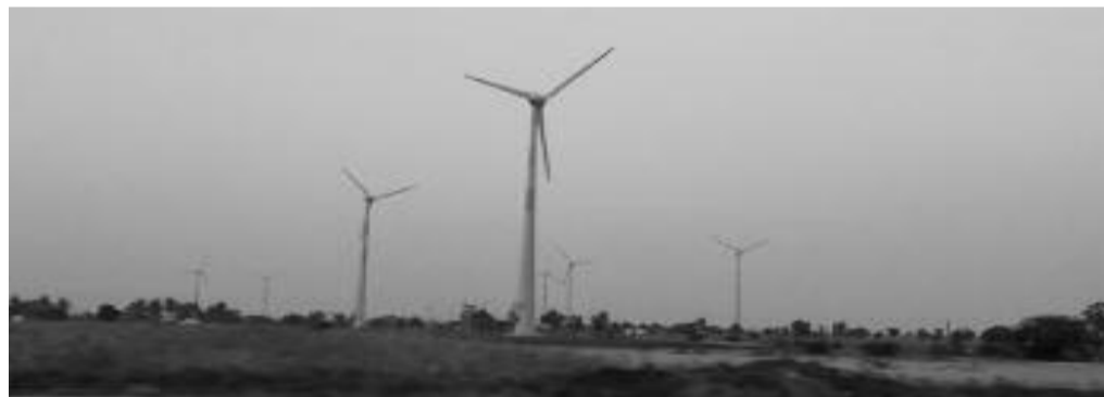
A windmill unit in Gadag which caters to power requirement of villagers. | BHAGYASRI
