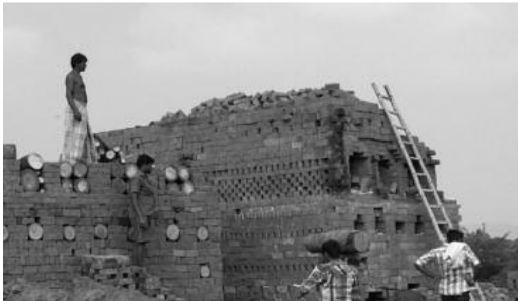
Overworked workers at the Brick Kiln hope for a better future.
